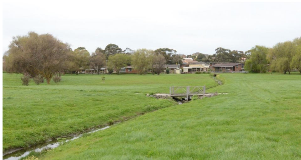
Figure 16 – Constructed, open drainage channel in St James Park
