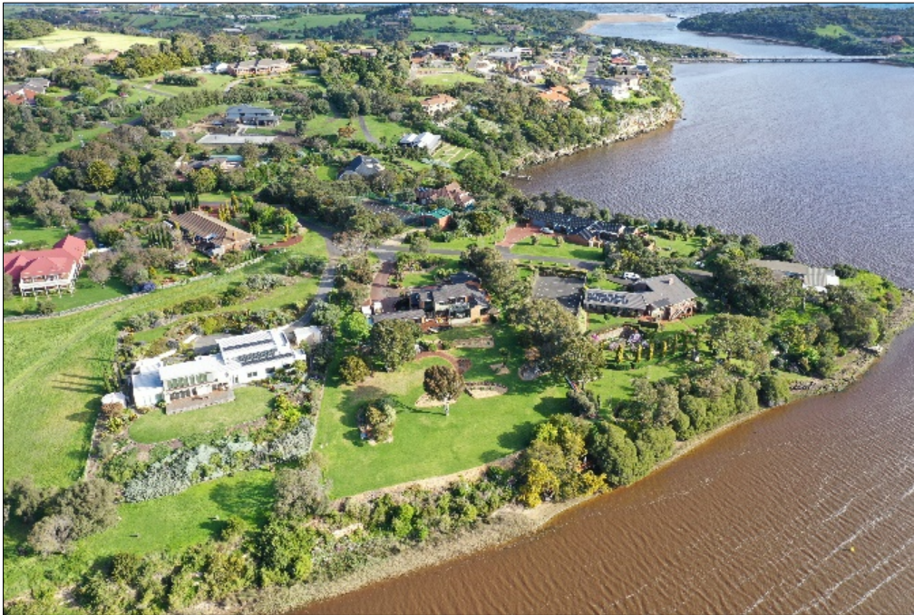
Figure 72 – Skeletal sandy loam soils within watercourse setbacks require careful monitoring of such systems within the Banksia Drive area.
