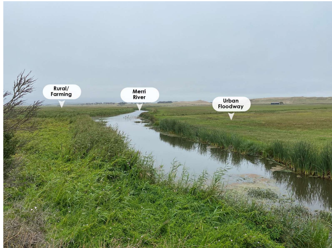
Photograph 12: View north-west from Crowes Bridge, Swinton Street
