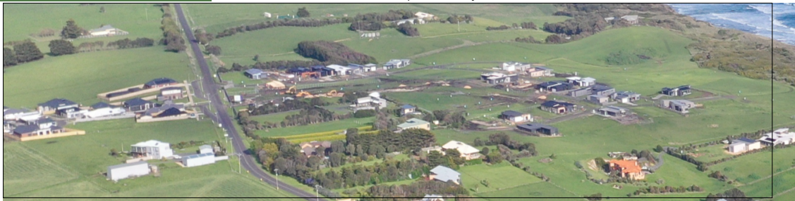
Figure 23 - Wannon Water has sewered two new estates within the Hopkins Point precinct providing a future connection framework for the area.
