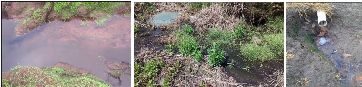
Figures 1-3 – Examples of failed and surface discharging wastewater systems.
