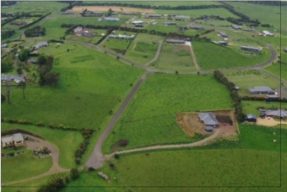
Figure 50 – Climery Crescent Woodford contains some slope-constraining lots managed via terracing, secondary treatment, and upslope diversion drainage.
