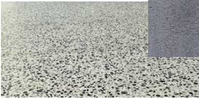
EXPOSED AGGREGATE FEATURE PAVING
