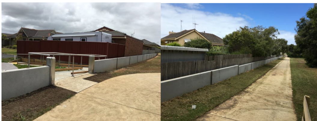
Figure 3. Constructed flood walls. (Source; Water Technology 2017).
