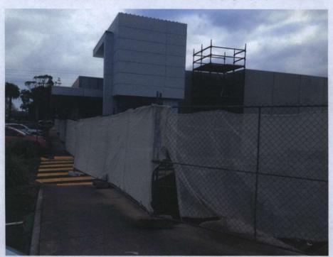
PHOTO 8 – Existing temporary construction fencing with weathered shade cloth to be replaced with new banner signage.
