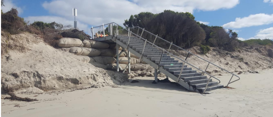
FIGURE 2-11 EROSION SCARP ALONG LADY BAY BEACH (PHOTOGRAPH TAKEN 16/04/19)
