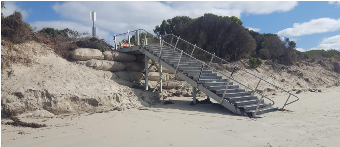
FIGURE 2-5 EROSION SCARP ALONG LADY BAY BEACH
