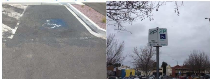
Figure 2: Line marking and signage renewal example
