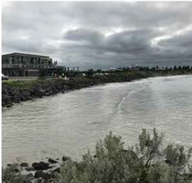
Rock work provides protection from coastal processes but also creates a buffer between pedestrian areas and the beach.
