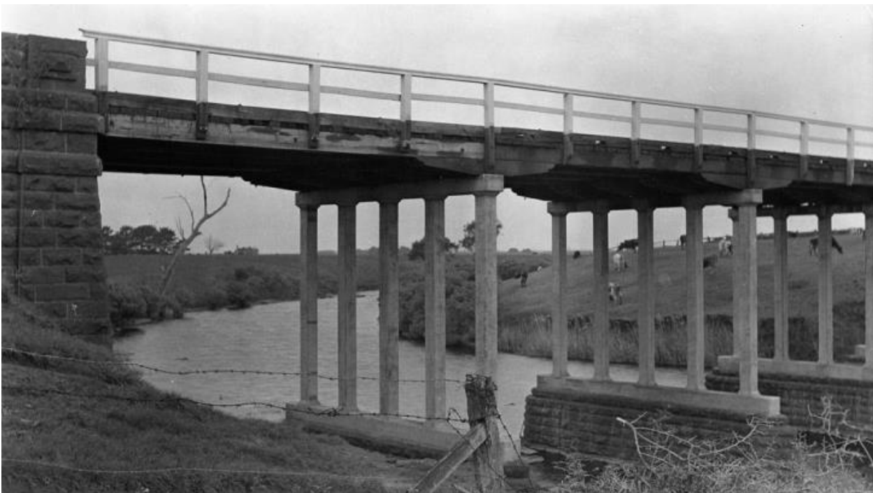
Photo: Pre-1937 showing concrete columns constructed on bluestone footings with timber beams and deck
