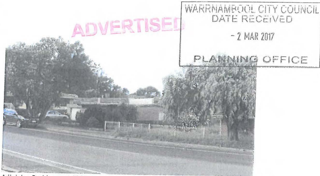
Adjoining Residence at 101 Merrivale Drive with low roof profile and parapet brick garage
