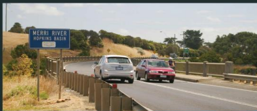
The bridge over the Merr River is narrow and unable to support fully loaded AB milk tankers which are integral to the South West dairy industry
