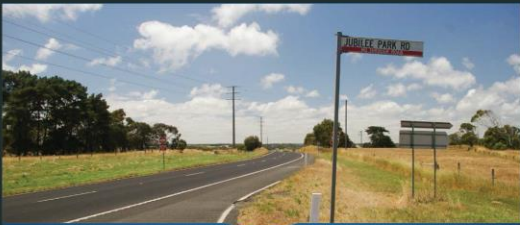
Deceleration lanes are required in the approaches to key intersections along rural sections of the highway including here at Jubilee Park Road
