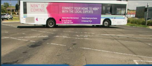
Pavement and road markings at Princes Highway-Gateway Rd intersection
