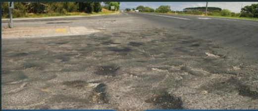
Safety and pavement improvements required at the intersection of Princes Highway and Garabaldi Lane, Allansford
