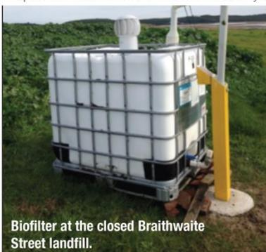
**Biofilter at the closed Braithwaite Street landfill.**
