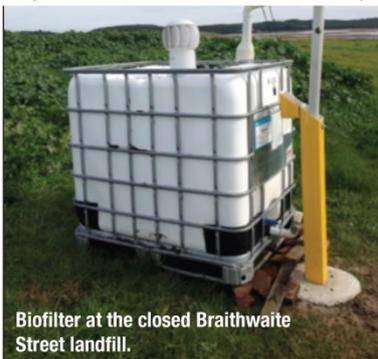
**Biofilter at the closed Braithwaite Street landfill.**
