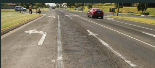
Increasing traffic loads have created challenges around maintenance of the road pavement
