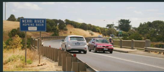
The bridge over the Merri River is narrow and unable to support fully loaded AB milk tankers which are integral to the South West dairy industry
