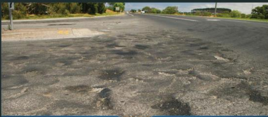
Safety and pavement improvements required at the intersection of Princes Highway and Garibaldi Lane, Allansford
