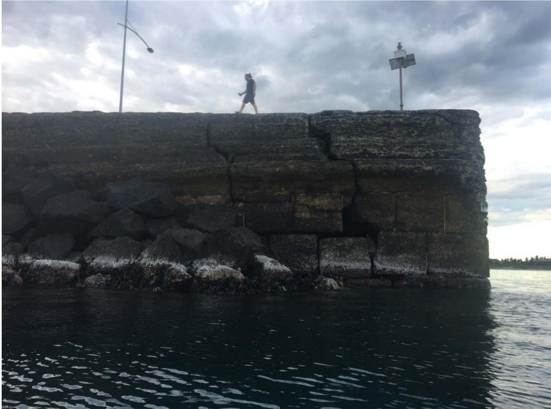
Figure 11 Armour Rocks at Breakwater Head
