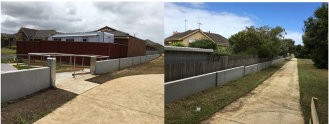
Figure 3. Constructed flood walls. (Source; Water Technology 2017).
