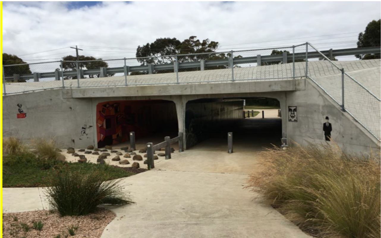
Figure 4. Constructed culverts under Mortlake Road. (Source; Water Technology 2017).
