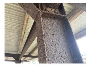
Facing E Portal column severely corroded.
