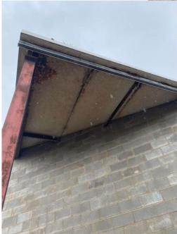
Photo 7: Corrosion of exposed column, purlins, bridging and soffit lining to dairy selling shed.
