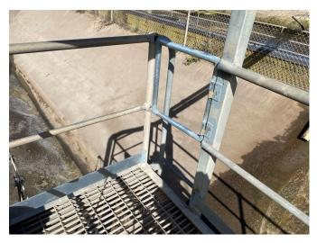
Photo 12: Gate at end of platform over west clarifying basin with no lock to prevent unauthorised access.
