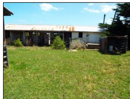
Plate 6: Milking shed in SU 2 – facing west (photo by M Reith 11/1/21)
