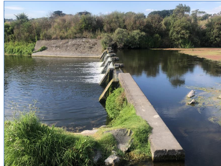
Figure 12 | View of Bromfield Weir looking north
