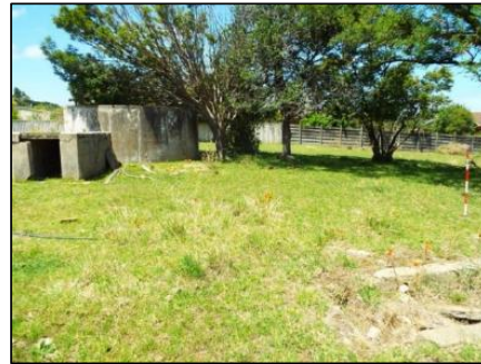
Plate 8: Concrete structures in SU 2 – facing east (photo by M Reith 11/1/21)
