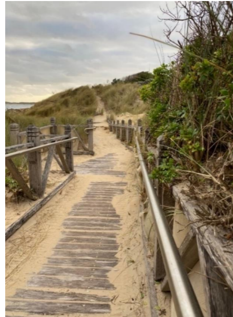
Figures 12: Sand build up on ramp (WCC126)
