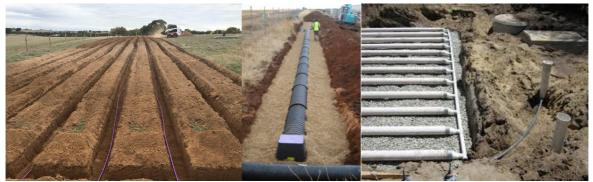
Figures 16-18: ETA beds can be used with septic tanks to reduce and concentrate affluent disposal area; another useful upgrade option for small lots and aging systems (Source: Hydroscape 2019, William Cromer 2019, Momington Peninsula Shire Council 2015).
