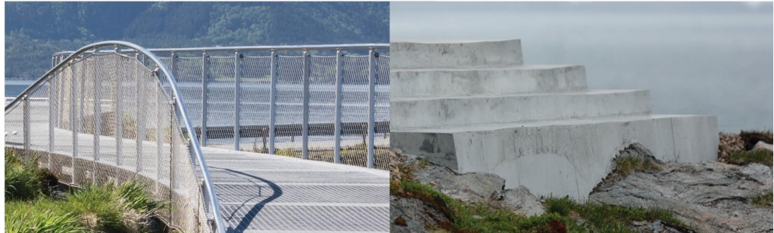
Steel - structural grade and hot dip galvanised as per AS/NZ 4680 for superior performance and powder coated for corrosive protection. Photo: Jarle Waehler Concrete - durable providing there is adequate cover to all reinforcement to prevent corrosion. Photo: Jarle Waehler
