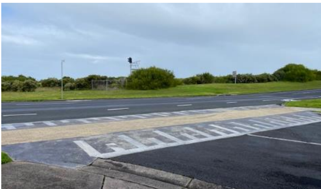
Photo 4: Raised threshold treatment – intersection of Merri Street and Annes Lane
